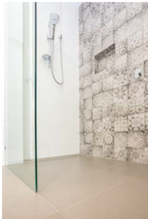
Image 6. Step-free shower with removable screen (Courtesy of Taylor'd Distinction)
