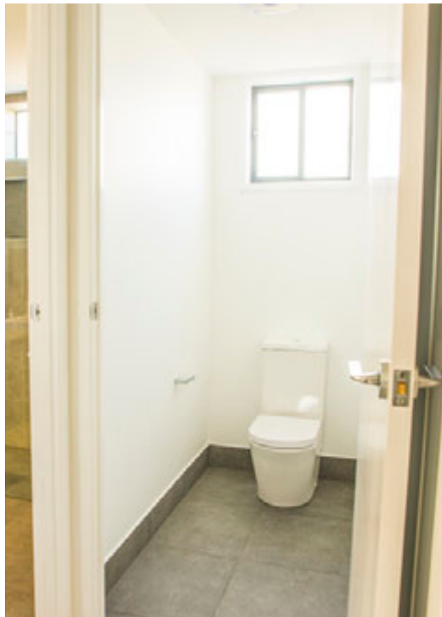
Image 5. Toilet at ground level with adequate space in front of the pan and either side of the toilet (Courtesy of Parent to Parent Assoc. QLD - P2P Housing Team)
